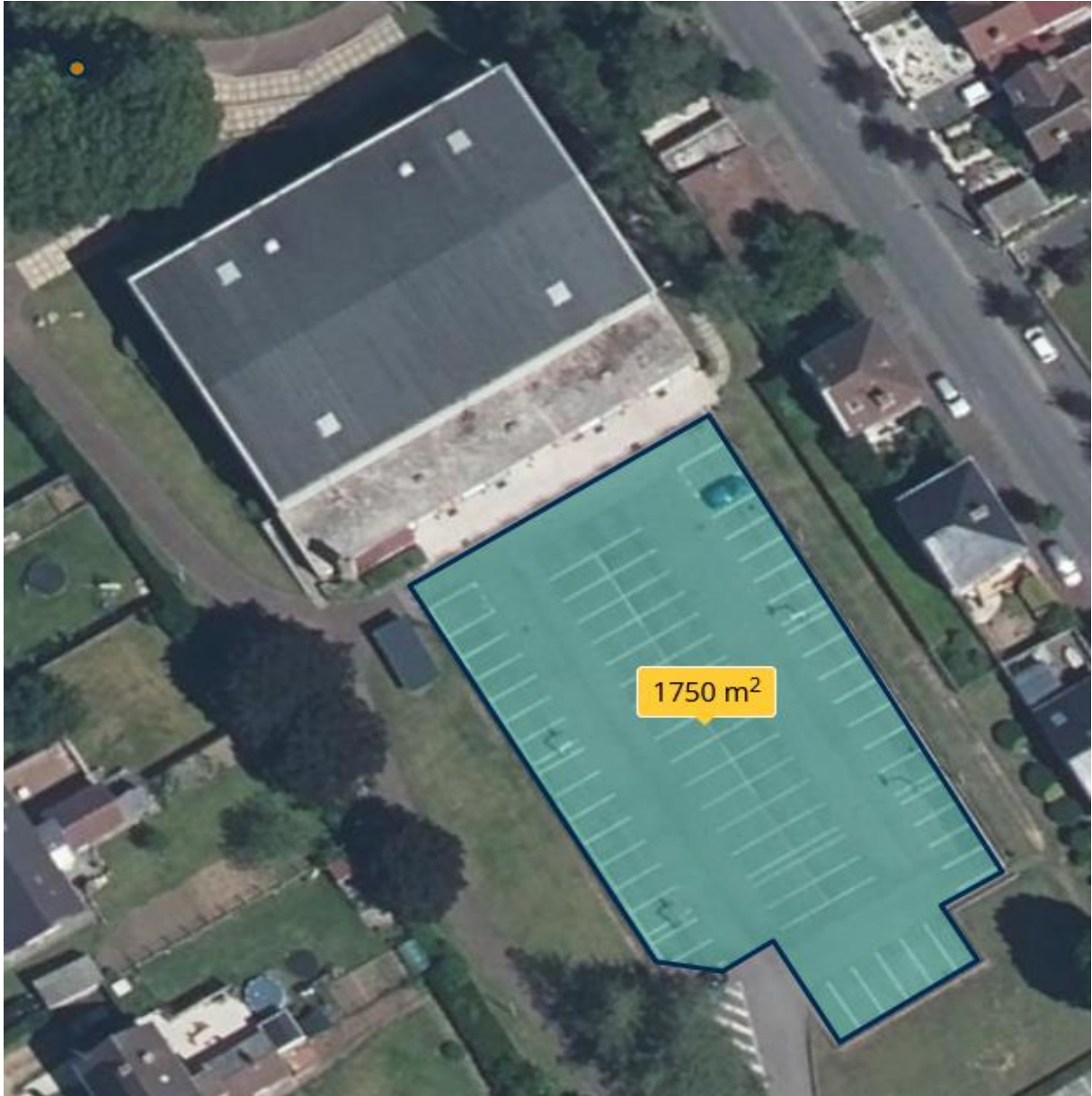
Parking Halle Vezillier-Descartes
